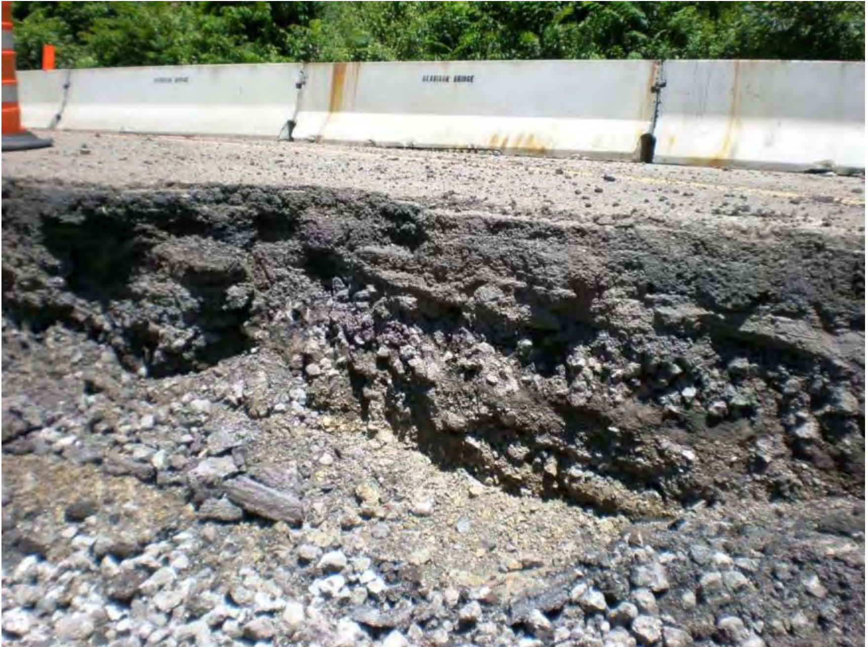
30 inches of pavement exposed
