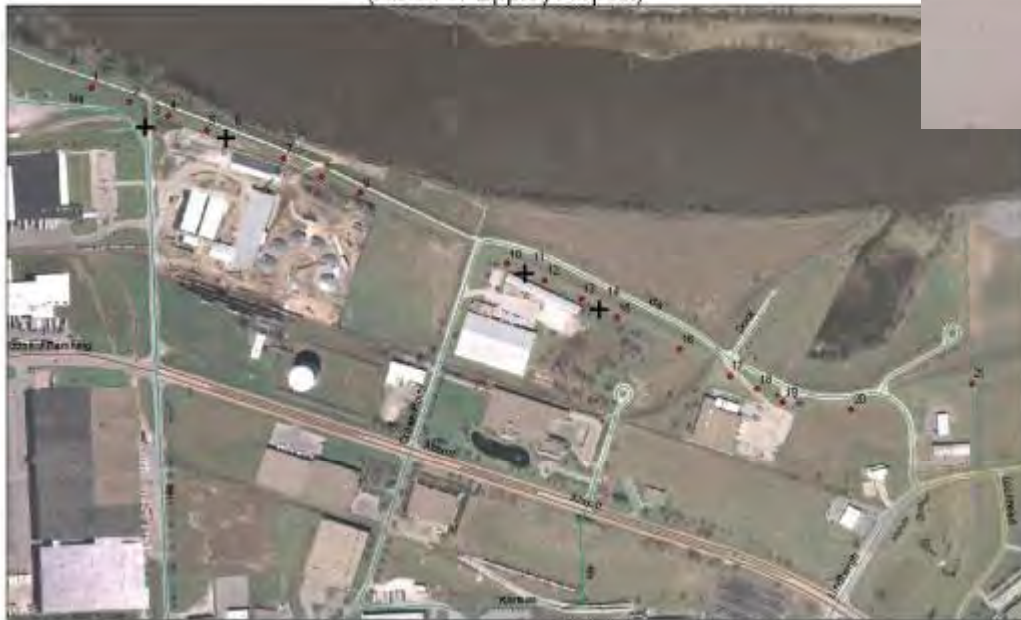
Levee Wells and Piezometers (North of Eppley Airport)
