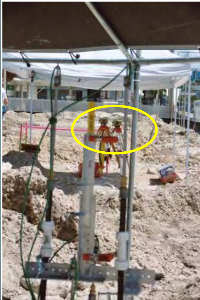
Leica digital levels monitor top of shaft directly
